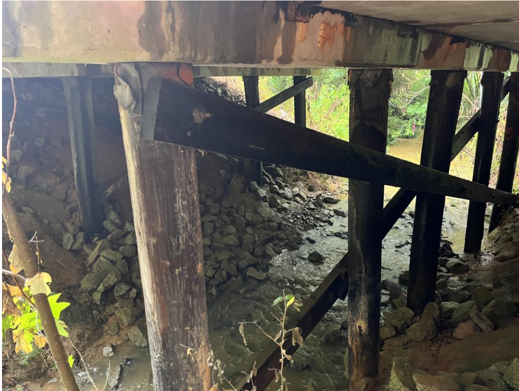
Photo 3 View of thin friction barrier between pier and pier cap.
