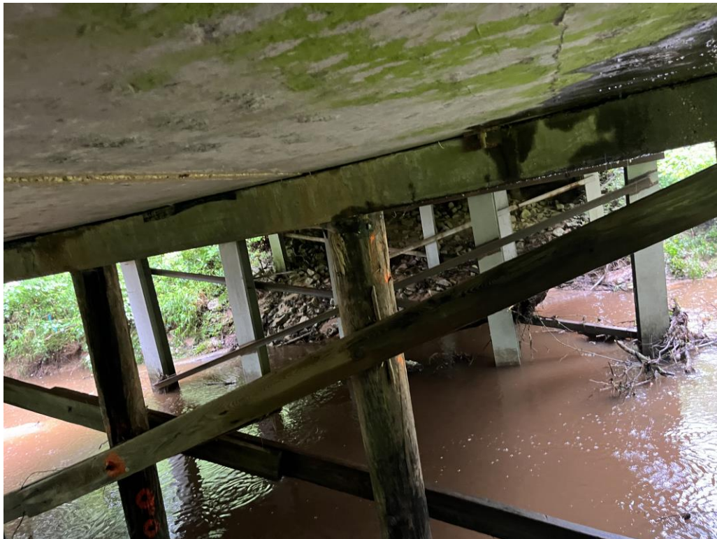
Photo 4 View of thin friction barrier between pier and pier cap.
