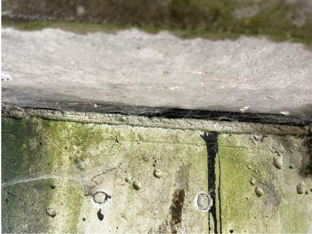
Photo 5 View of thick friction barrier in between pier cap and decking.
