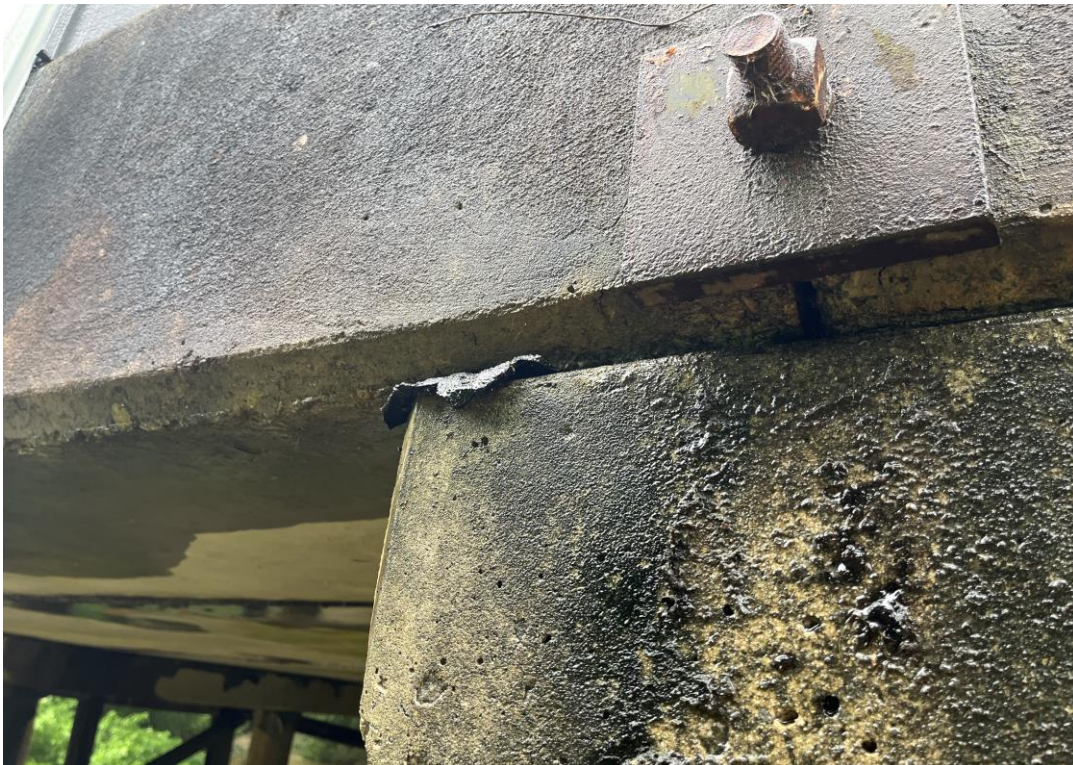
Photo 4 View of thick friction barrier between pier cap and decking and orange metal bracket.
