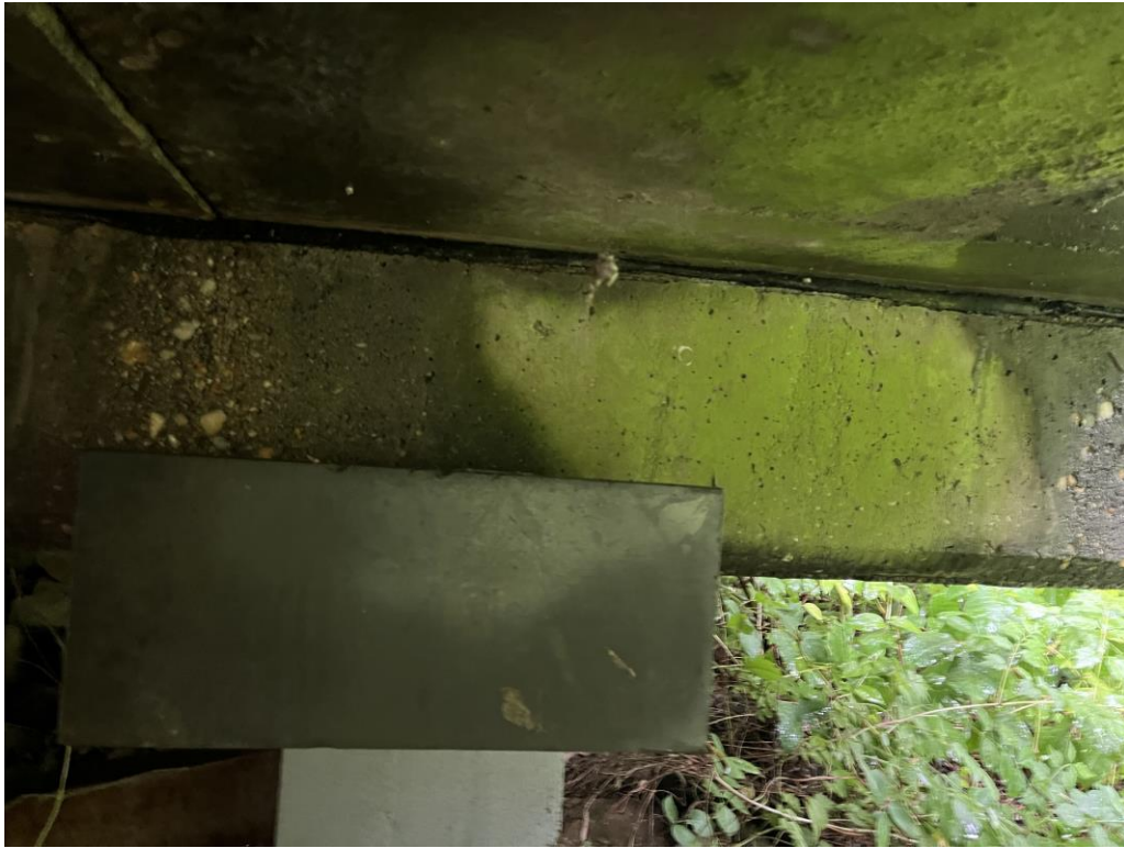
Photo 5 View of the thick friction barrier in between pier cap and decking.
