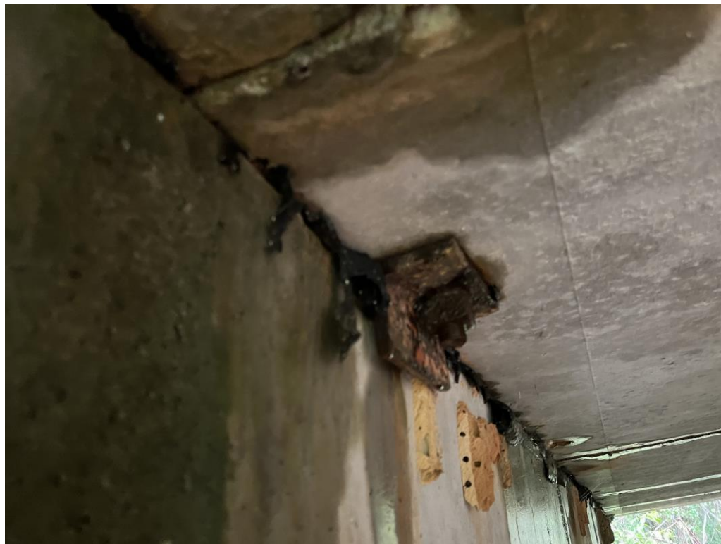
Photo 4 View of thick friction barrier between pier cap and decking and orange metal bracket.
