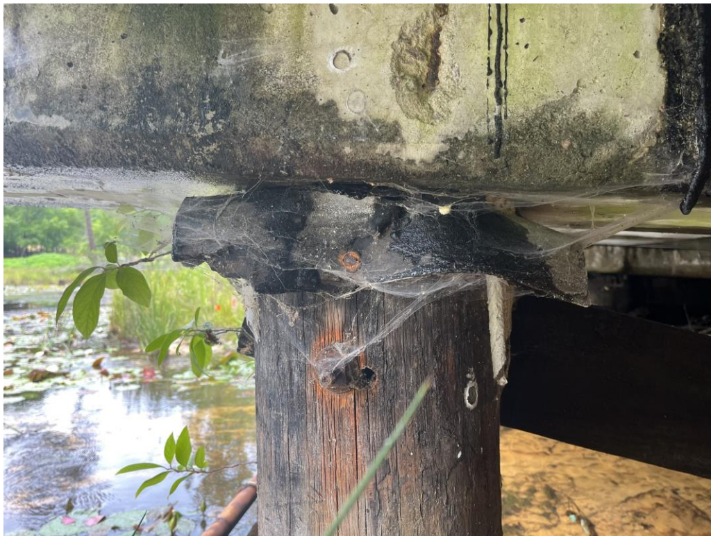
Photo 4 View of thin friction barrier in between pier and pier cap.
